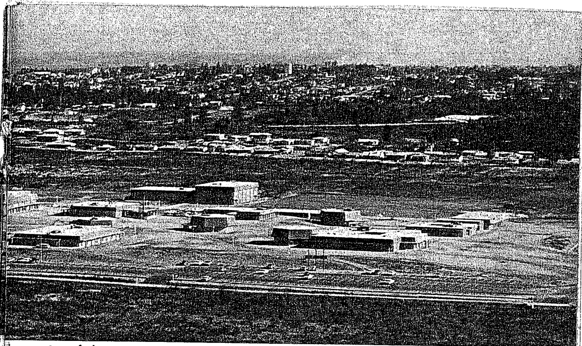
center of the campus is the Pearl A. Wanamaker Library and Instructional Resource Center. For more information on the college's physical facilities see Page 20 and the map inside the back cover.—Photo by Buz Demarest
